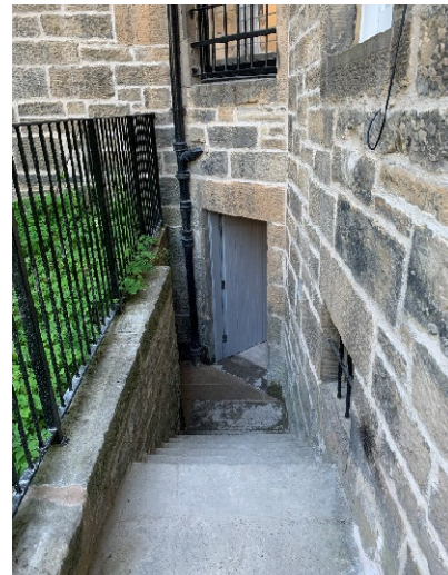
New balustrade, slabs and decoration
