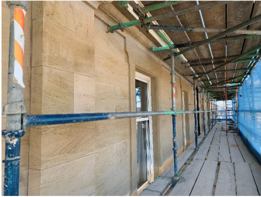
Stone replacement to front elevation
