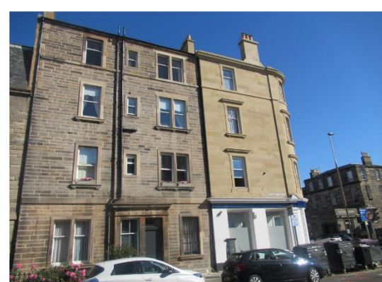
West elevation upon completion
