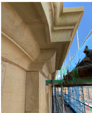
New stone cornice
