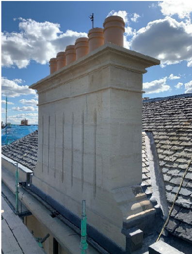
New stone wallhead chimney
