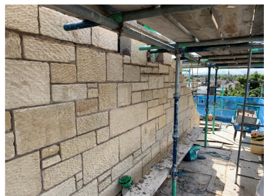
Build-up of gable chimney
